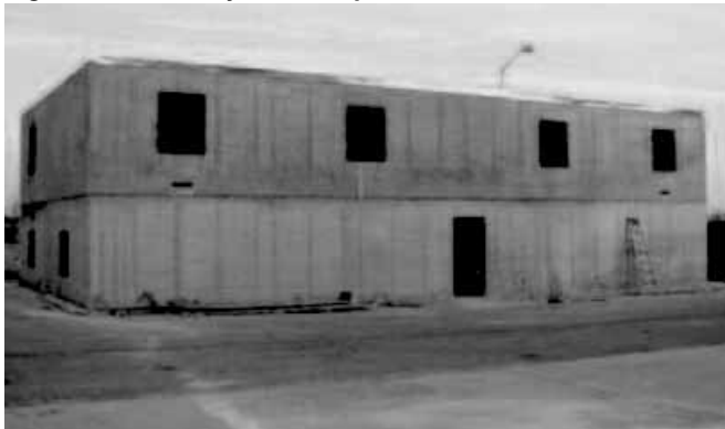
Figure 1: Two-Story Burn Prop
